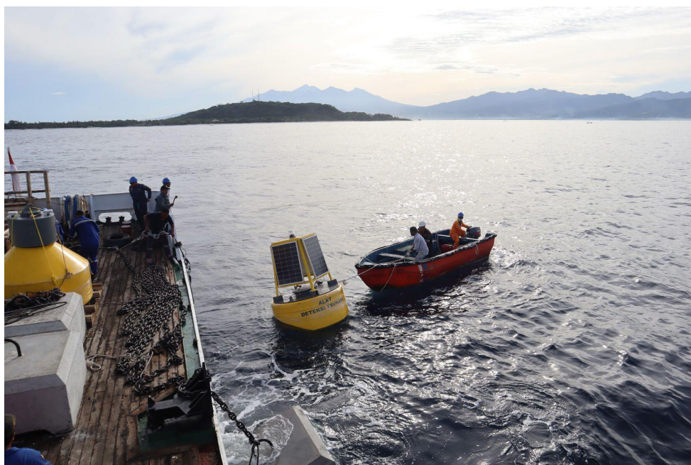
Photo 2. Illustration of the 2021 installation of a buoy-based Coastal Acoustic Tomography system on the eastern coast of Bali, implemented under the Indonesia Tsunami Early Warning System program (Source: Agustan, 2021).
